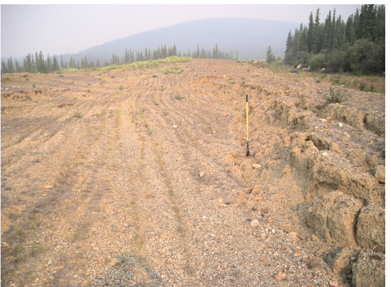
View northwest along the old Alaska Highway route, showing damage that occurred as a result of mass movement associated with thawing permafrost. Road was rerouted in 2004. (Photograph taken 08/10/2009 by R.D. Reger.)
