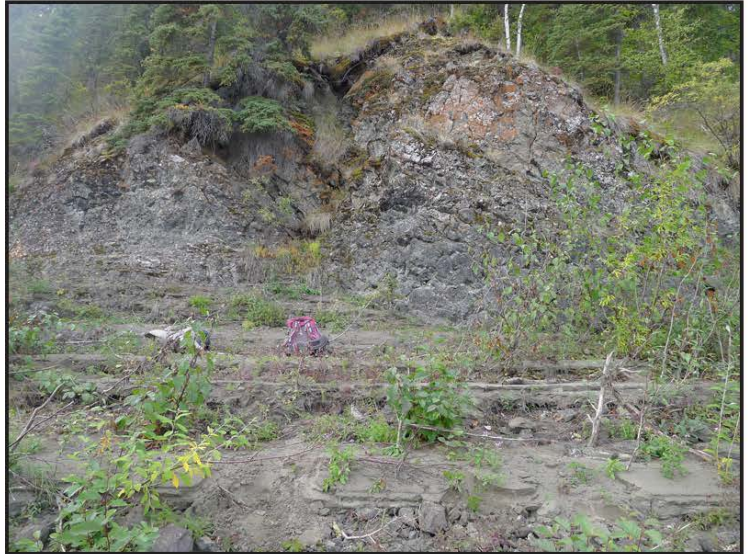
A13. Station 11 joint sets, between 625 and 675 feet east of the Yukon River bridge.
