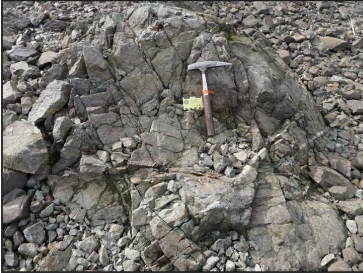
A14. Station 12 joint sets, between 850 and 900 feet east of the Yukon River bridge.
