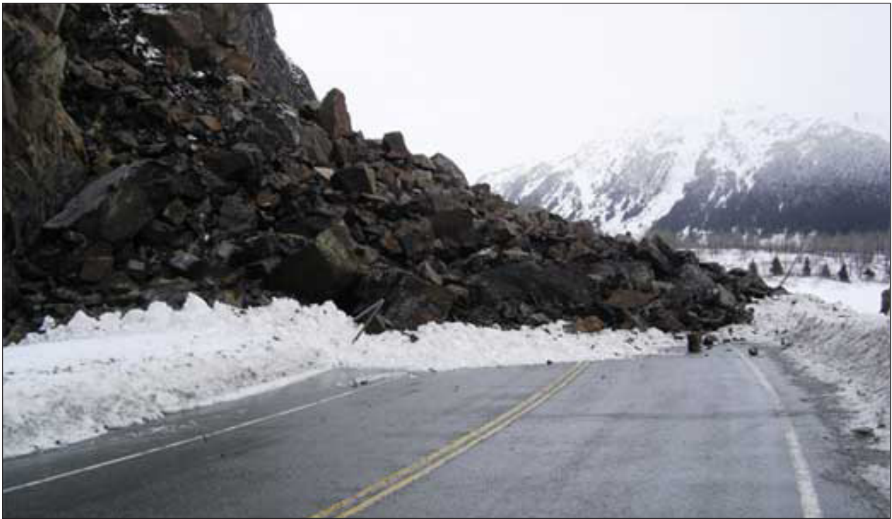
Figure 9. Rockfall debris on the Portage Glacier Highway, April 2009. Photo courtesy of the Alaska State Troopers.
