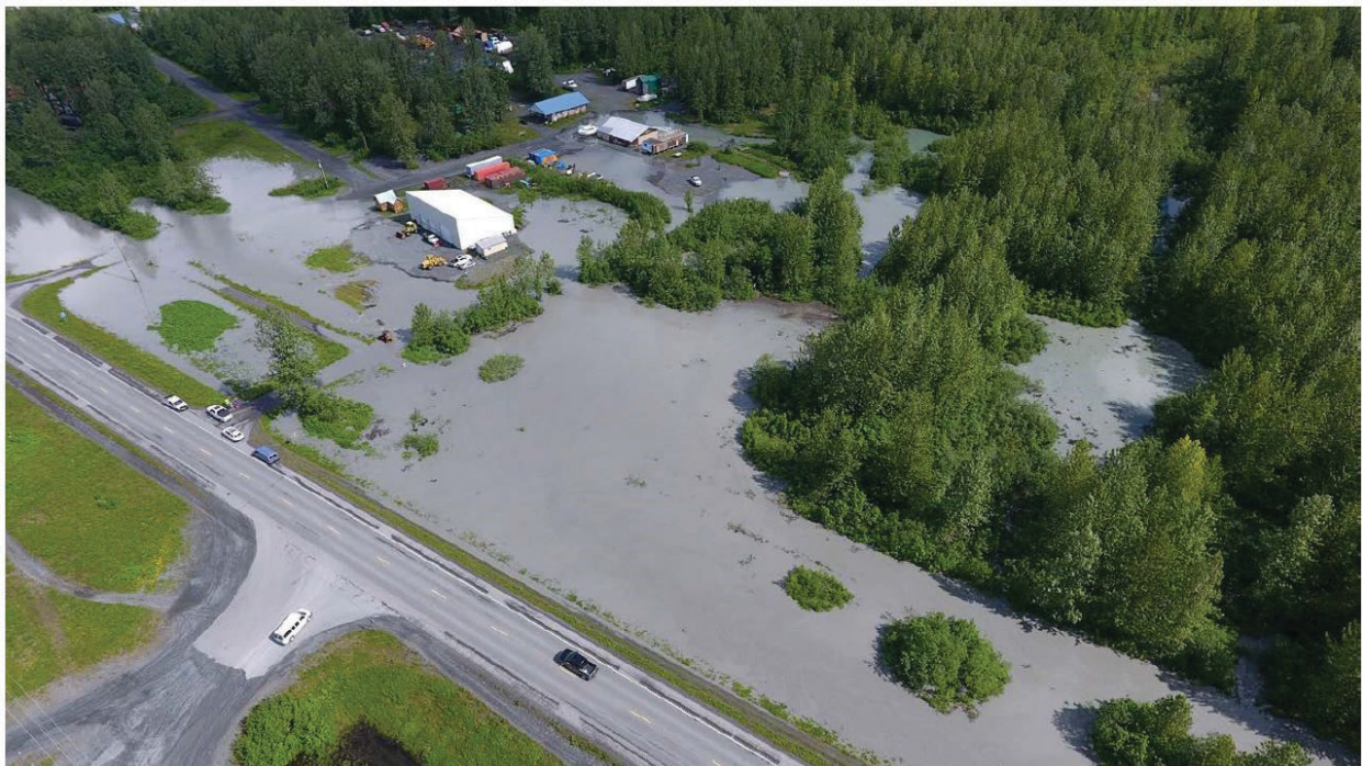
Figure 7. Flooded area near 9 th Street in Valdez (City of Valdez, written commun., June 2018).
